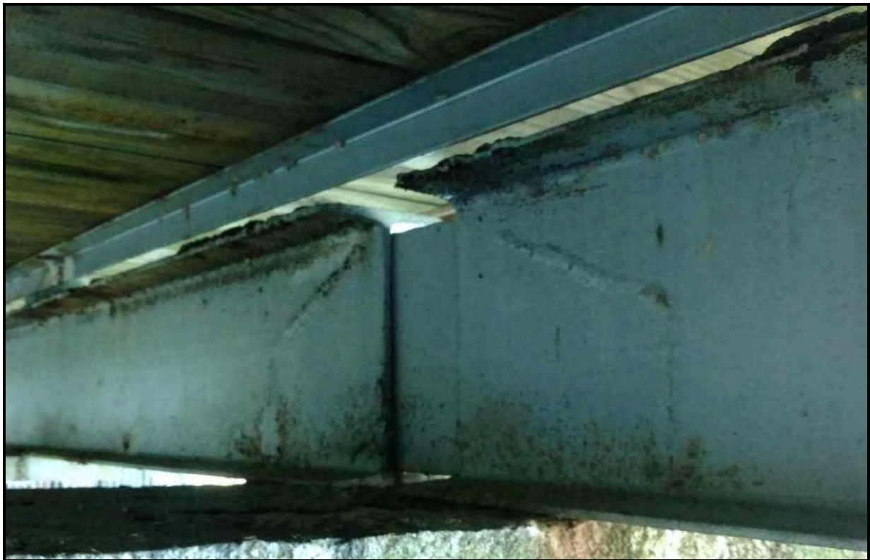
Photograph 30: Back side of typical bridge girder to bridge girder connection.
